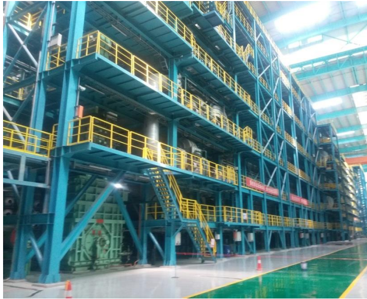
External view of Continuous Annealing and Processing Line (C.A.P.L.™) at Anyang Iron & Steel Co., Ltd.
