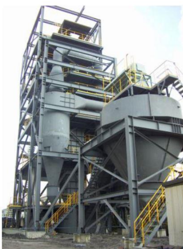
[Photo] Exterior of full-scale prototype
