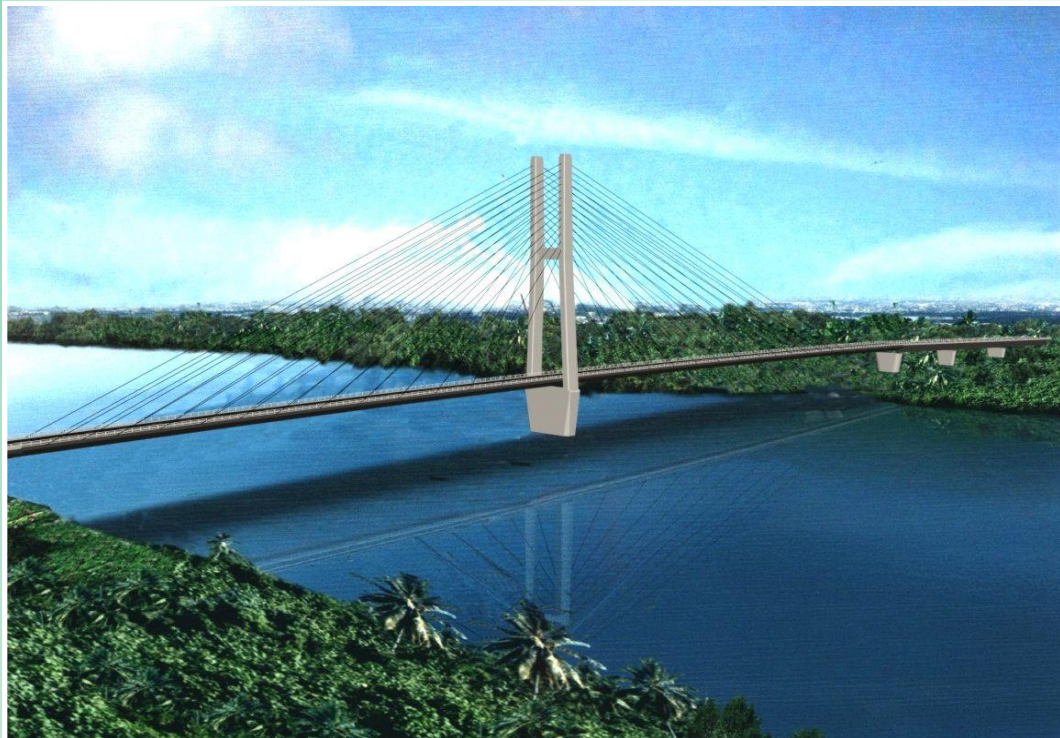
2 nd Magsaysay Bridge and City Bypass Road Project
