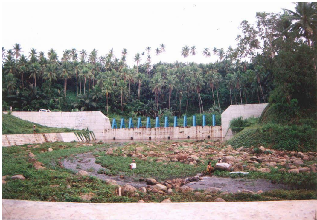
Slit Dam Project
