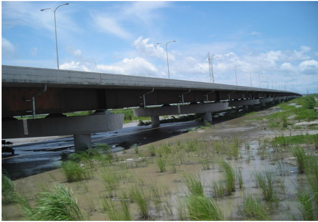
Subic-Clark-Tarlac Expressway Project Package 2
