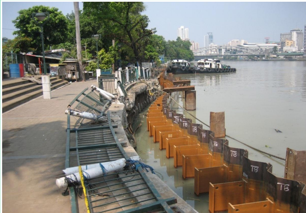
Steel Sheet Pile
