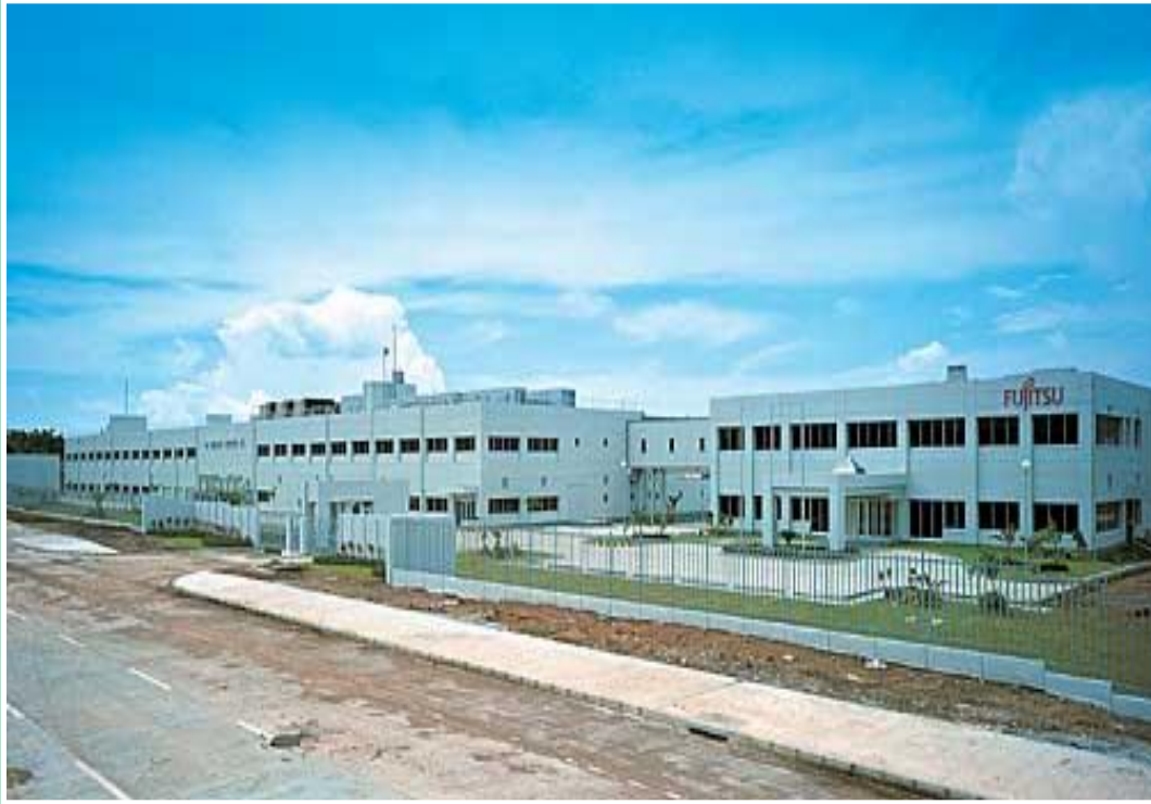
Fujitsu Factory Building II Project
