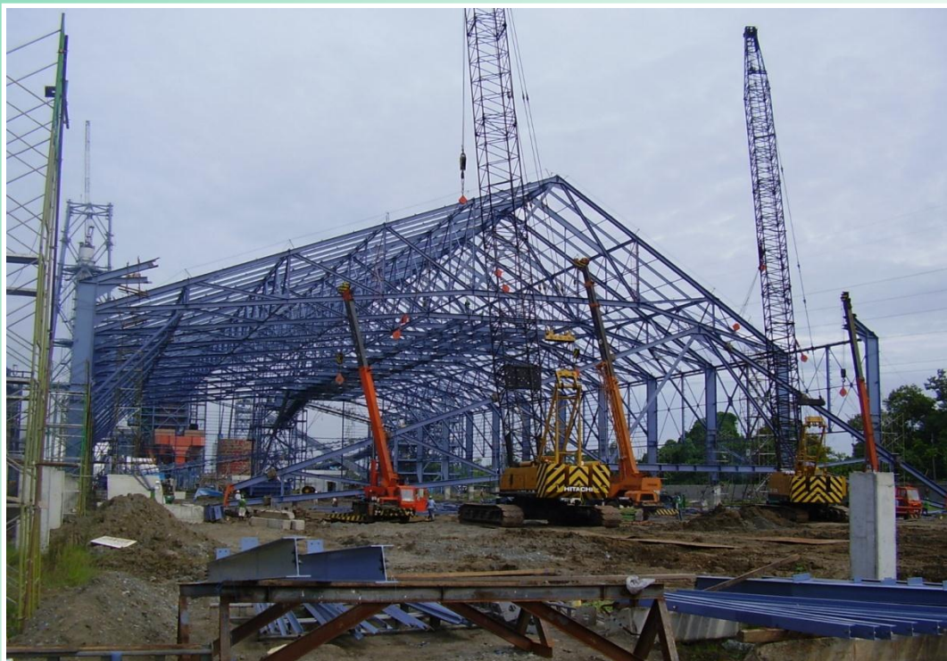
Cagayan de Oro Power Plant Project
