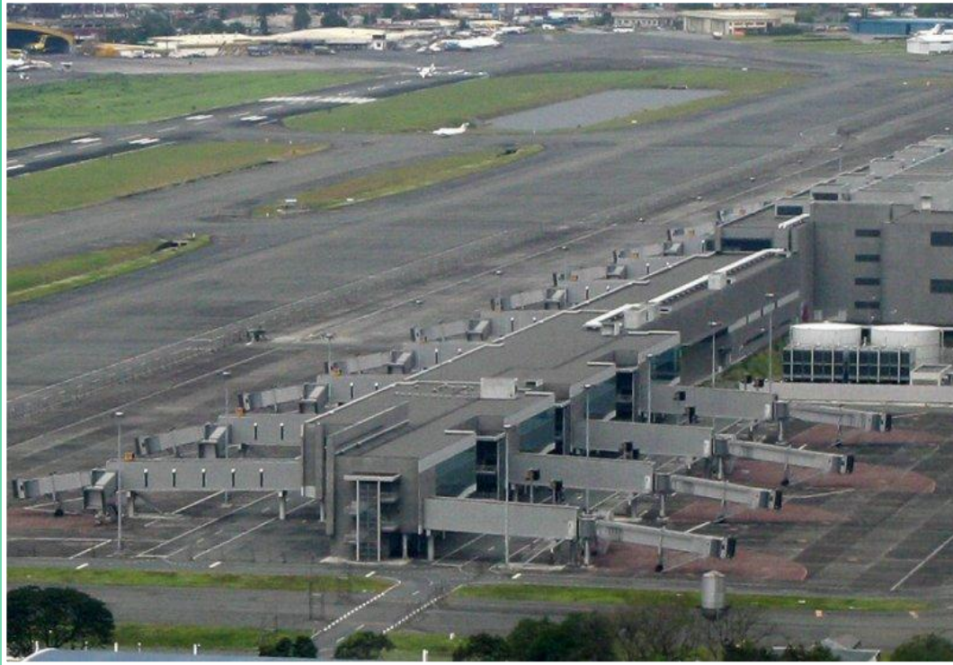
NAIA IPT3 Airport Project
