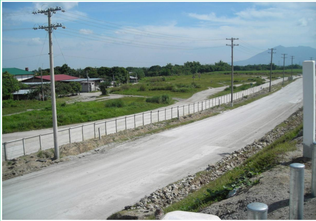
Subic-Clark-Tarlac Expressway-Fencing Project Package 2
