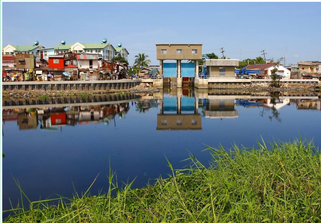
KAMANAVA Flood Control Construction Project
