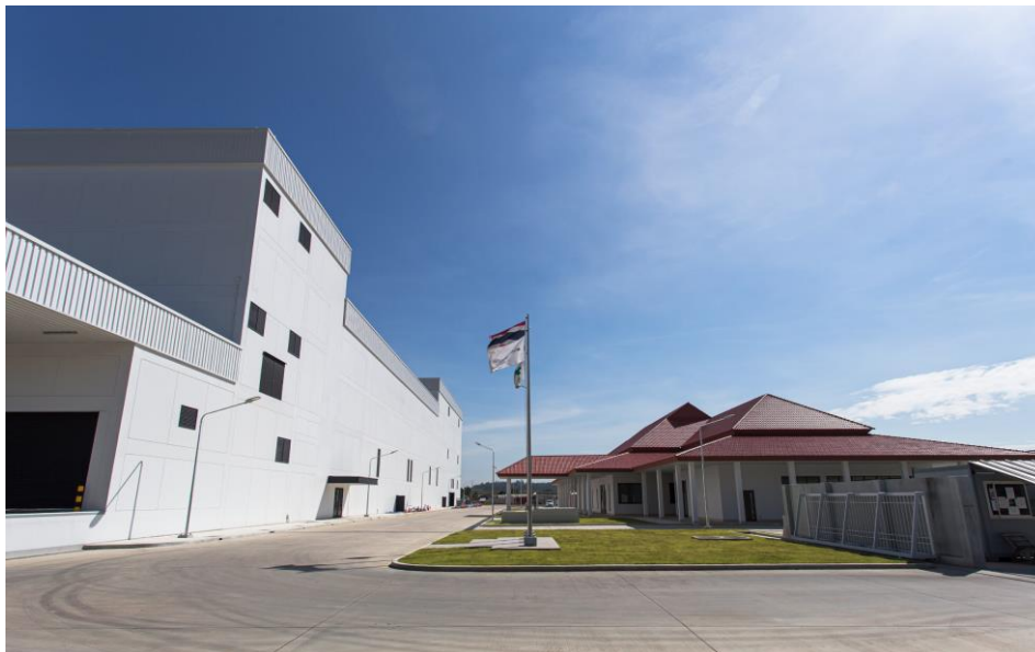
[The structural protein plant constructed by Spiber]
