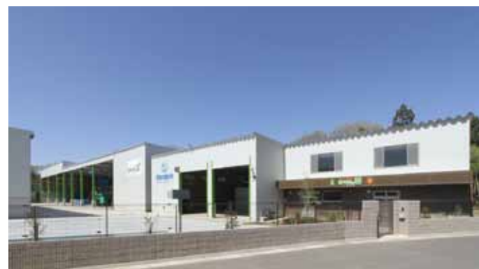
Intermediate Processing Facility Shiroi City, Chiba: 3,700m 2
