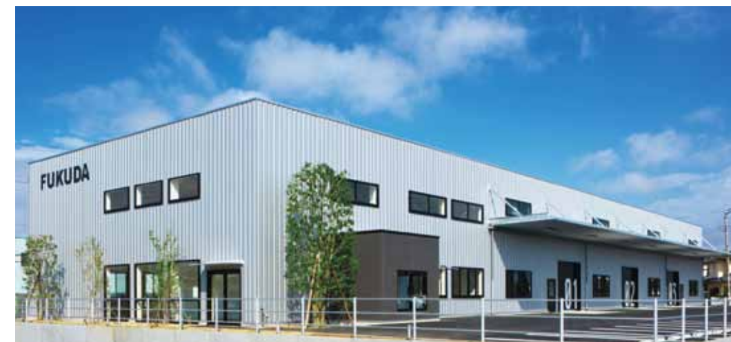
Logistic Center/ Office Hitachinaka City, Ibaraki: 1,400m 2 Apparel manufacturing and sales company head office and logistic center. Both design and economic efficiency are achieved.
