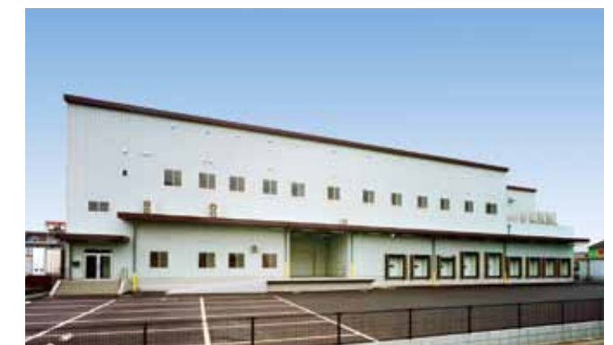
Refrigerator and Freezer Facility Fukuoka City, Fukuoka: 3,700m 2
