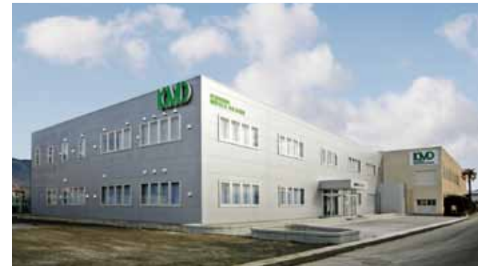
Office for an Electronic Components Manufacturing Company Date-gun, Fukushima: 1,300m 2
