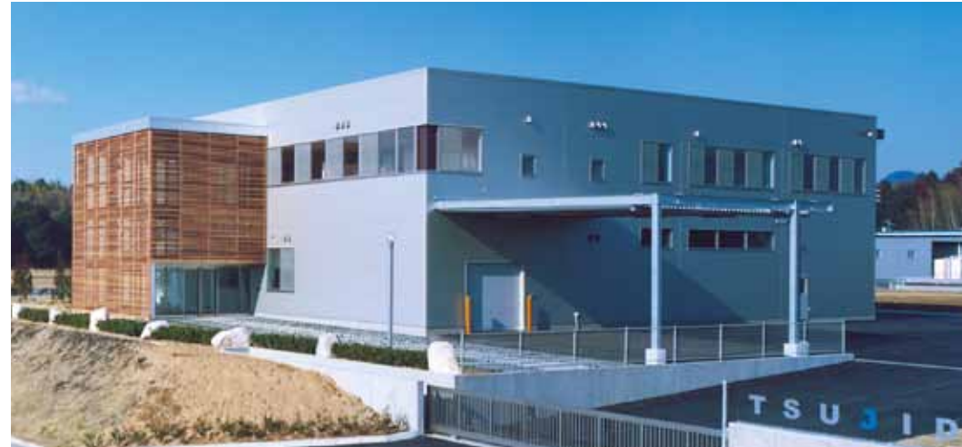
Storage Facility and Office
