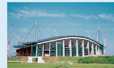
2000 Exposed Braces with Cast End Connections Toyota Stadium, Aichi
