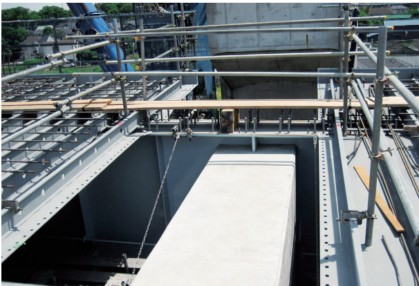
図24 中間支点落込みパネル箇所 Fig. 24 Adjust panel at an intermediate support
