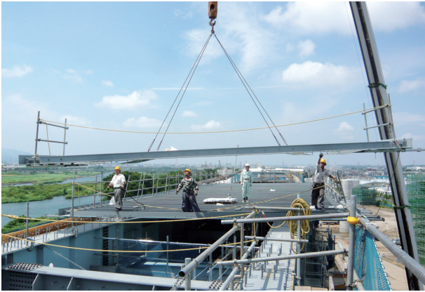
図22 床版パネル架設状況 Fig. 22 Erection of a floor panel
