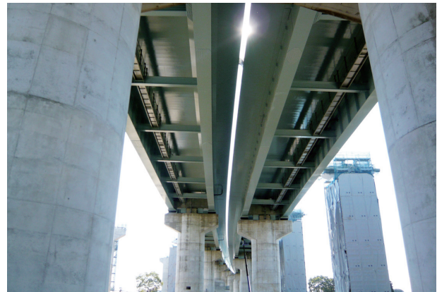
図27 完成写真 Fig. 27 General view of finished work
