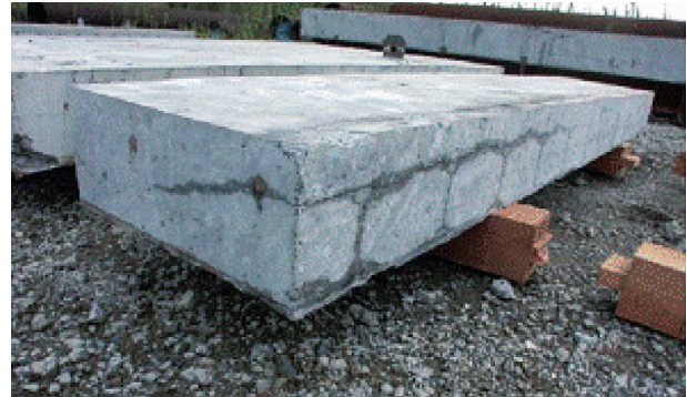
図8 輪荷重走行試験後の供試体切断状況 Fig. 8 Cutting plane of the specimen after wheel tracking test
