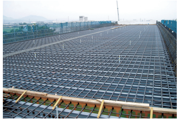
図25 鉄筋配筋状況 Fig. 25 Arrangement of reinforcement
