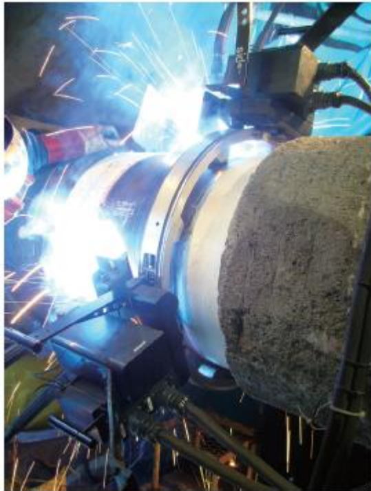
Fig. 6: Welding of pipelines using RAIDEN (photo)
