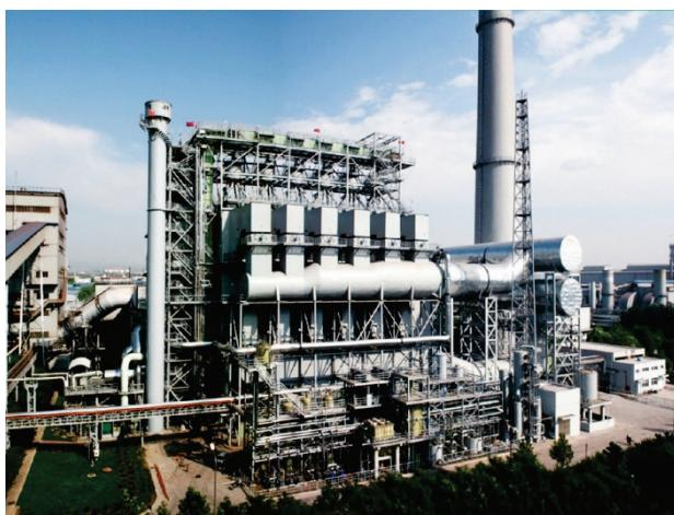
Figure 5 DDDS at Chinese steel company TISCO (commenced operation in 2010)
