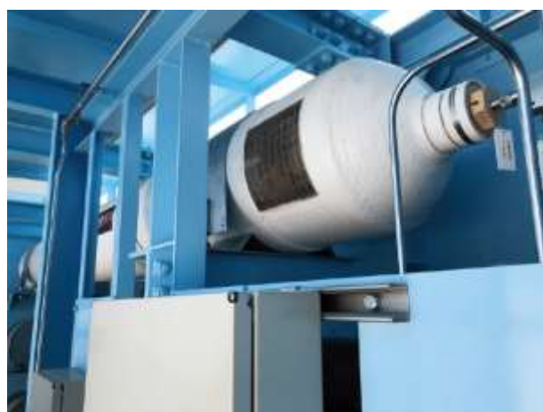
Figure 1 Installed FIBA type 2 pressure vessel
