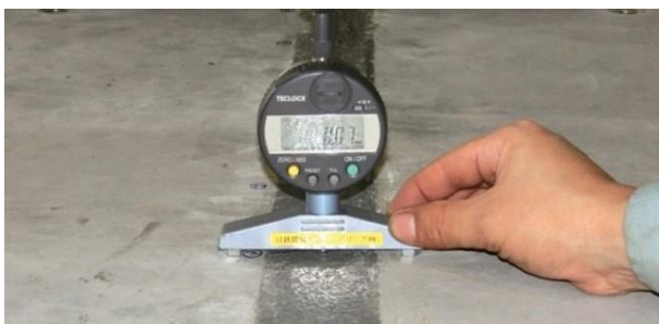
Fig. 6 Appearance of Measuring Settlement
