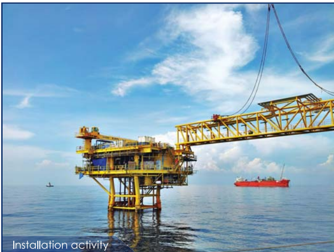
Installation activity by NSENGI Kuroshio
