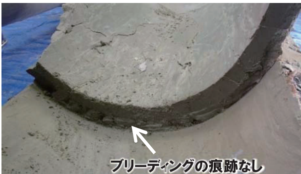
図14 充填完了状況(円筒状鋼製型枠底部) Fig. 14 View of the hardened full scale test body
