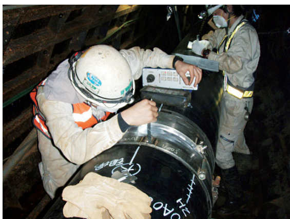
図11 配管芯出し状況(写真) fig.11 Operation of pipeline centering (Photo)
