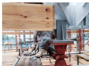
図16 鉄骨仮受(写真) Fig. 16 Temporary support of steel member (Photo)
