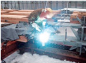
a) 鉄骨現場溶接 a) Site welding
