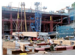
図15 荷下しと仮置(写真) Fig. 15 Unloading and temporary installation (Photo)
