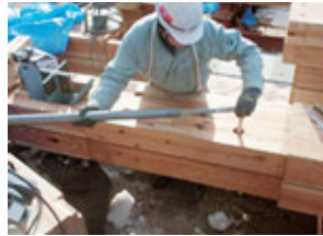
b) 集成材取付 b) Installing of glulam timbers
