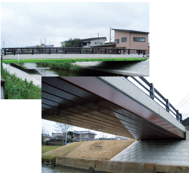
図1 角太橋写真 Fig. 1 appearance of KAKUTABASHI
