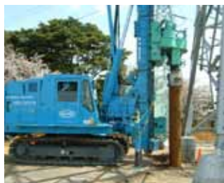
写真3 小径施工 Photo.3 Construction machine (small size)
